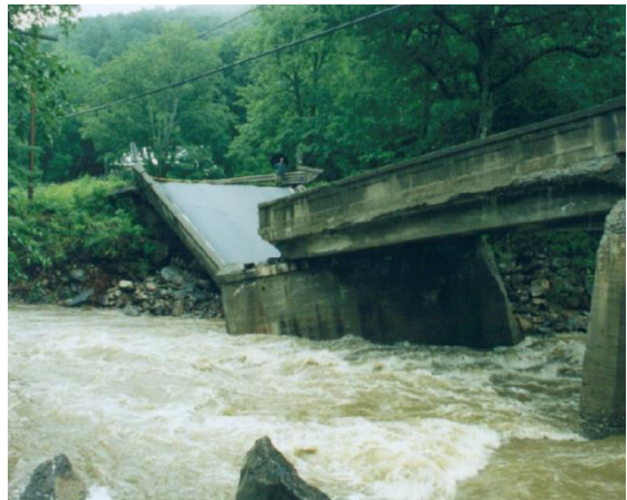
Fig. 1: Flood Damage in Bristol
