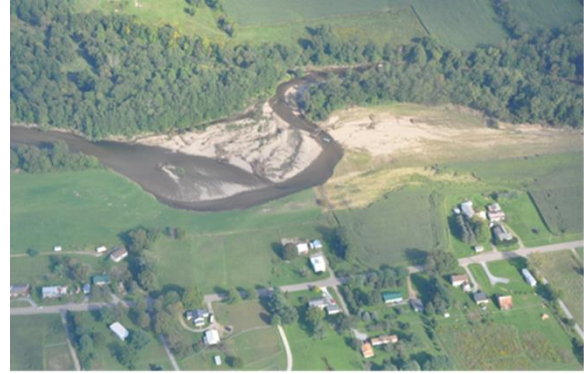
Fig. 2: Bird's eye view of site
